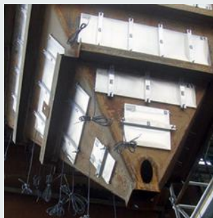
Hopper Heater Installation
